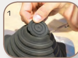
1 Choose the pipe opening and trim the sleeve
