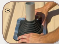
3 Slide the boot over the pipe and form to the roof profile
